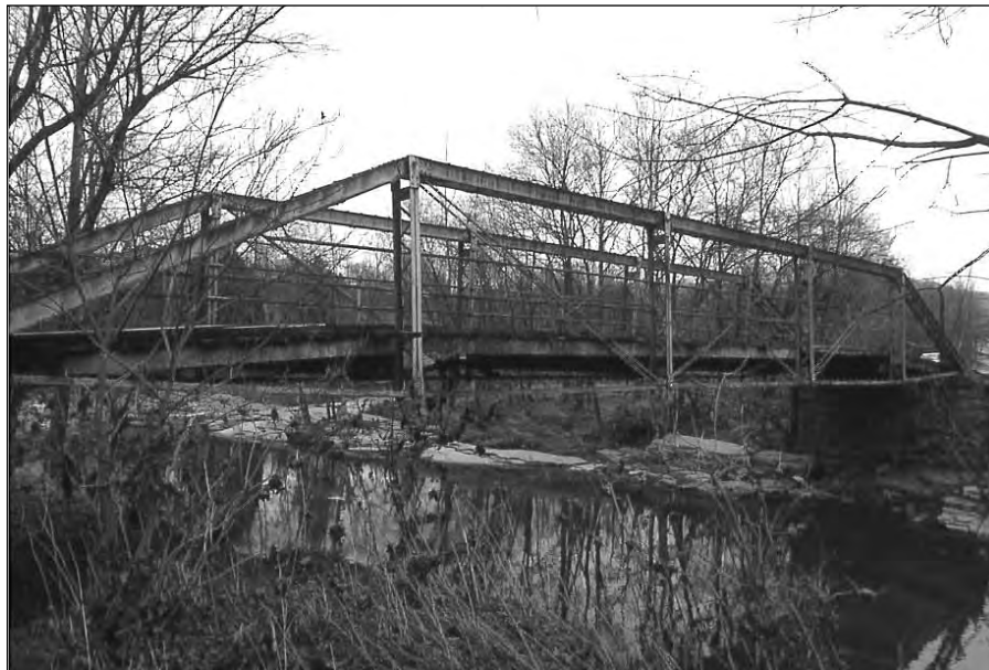
Figure VII-06: The Buena Vista Ford Bridge spanning Lick Creek Smith County (#56, 80- A0206-00.47) is an atypical Pratt truss with fishbellied bottom chord built in 1907 by the W.T. Young Bridge Company (above). In 1986 TDOT removed the truss span (top next page) and lifted it off its original abutments and moved it on a truck to Loudon County (middle next page). This view shows it on a tandem truck negotiating a curve in rural Smith County. The City of Loudon renovated the bridge for pedestrian use on a city trail (bottom next page).
