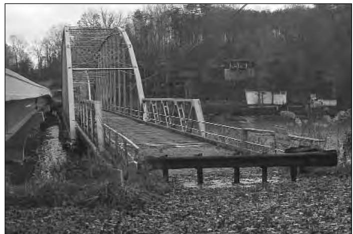
Figure VII-02: Photograph of the Rock Island Bridge in Warren County (#112, 89-04261-11.60).
