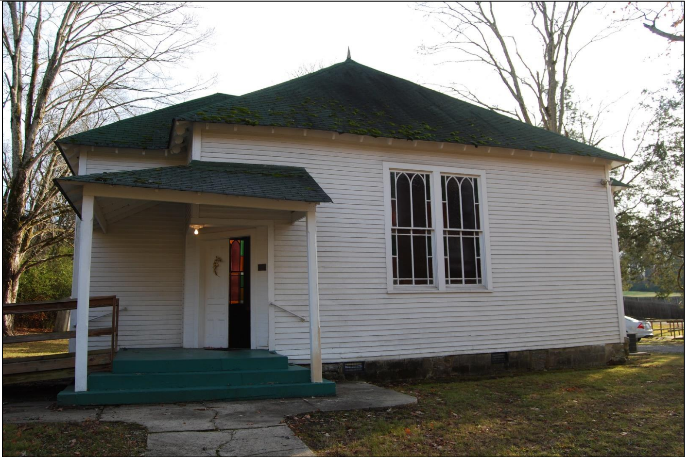
Figure 9: Ebenezer Cumberland Presbyterian Church, 2019. From National Register Nomination.
