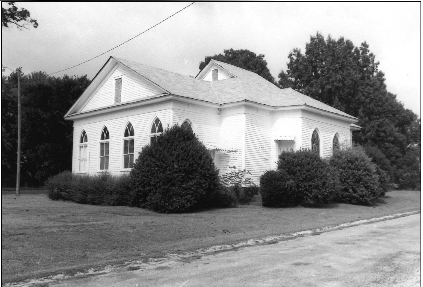
Figure 2: September 1976 Survey Photo of the Woodlawn Baptist Church, showing the west and south elevations. From the Tennessee Historical Commission Survey Files.
