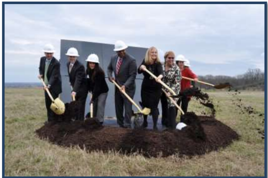
Above, the ground breaking moment for the Music City Solar Array Project on March 5 th 2018.
